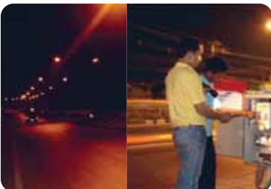
Lighting System - Department of Highways
